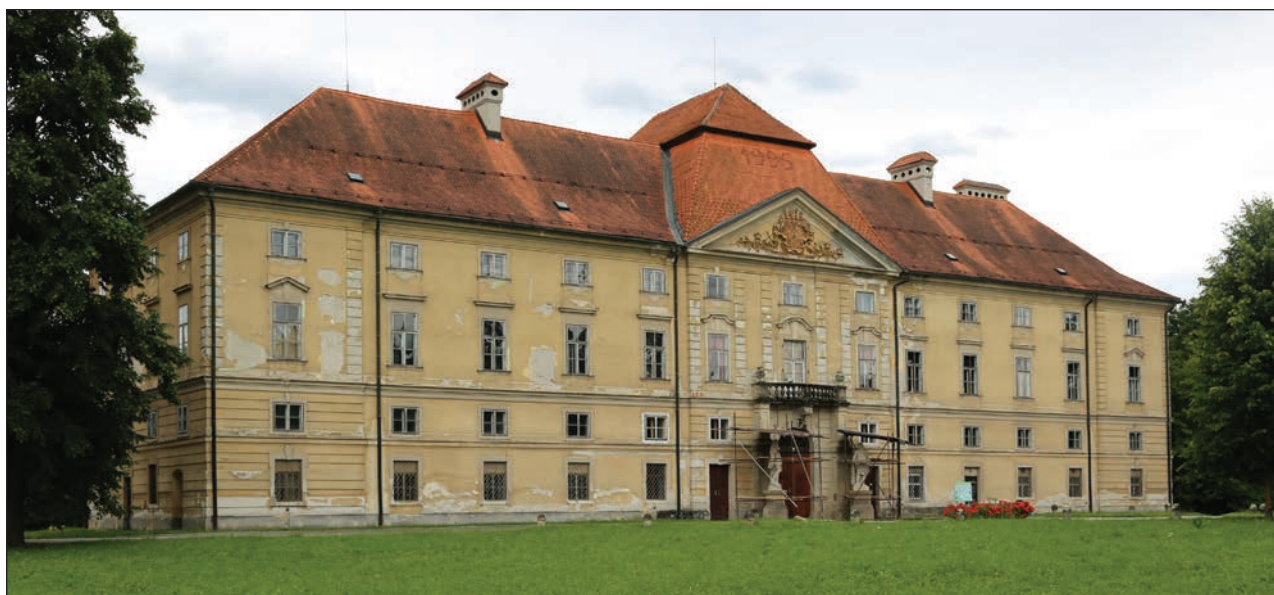
Figure 1: Main facade of the Novo Celje manor, 2020 (Photo: I. Sapač).
