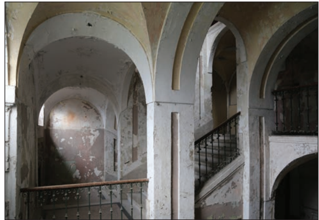
Figure 10: The main staircase in the Novo Celje manor, 2022 (Photo: I. Sapač).
