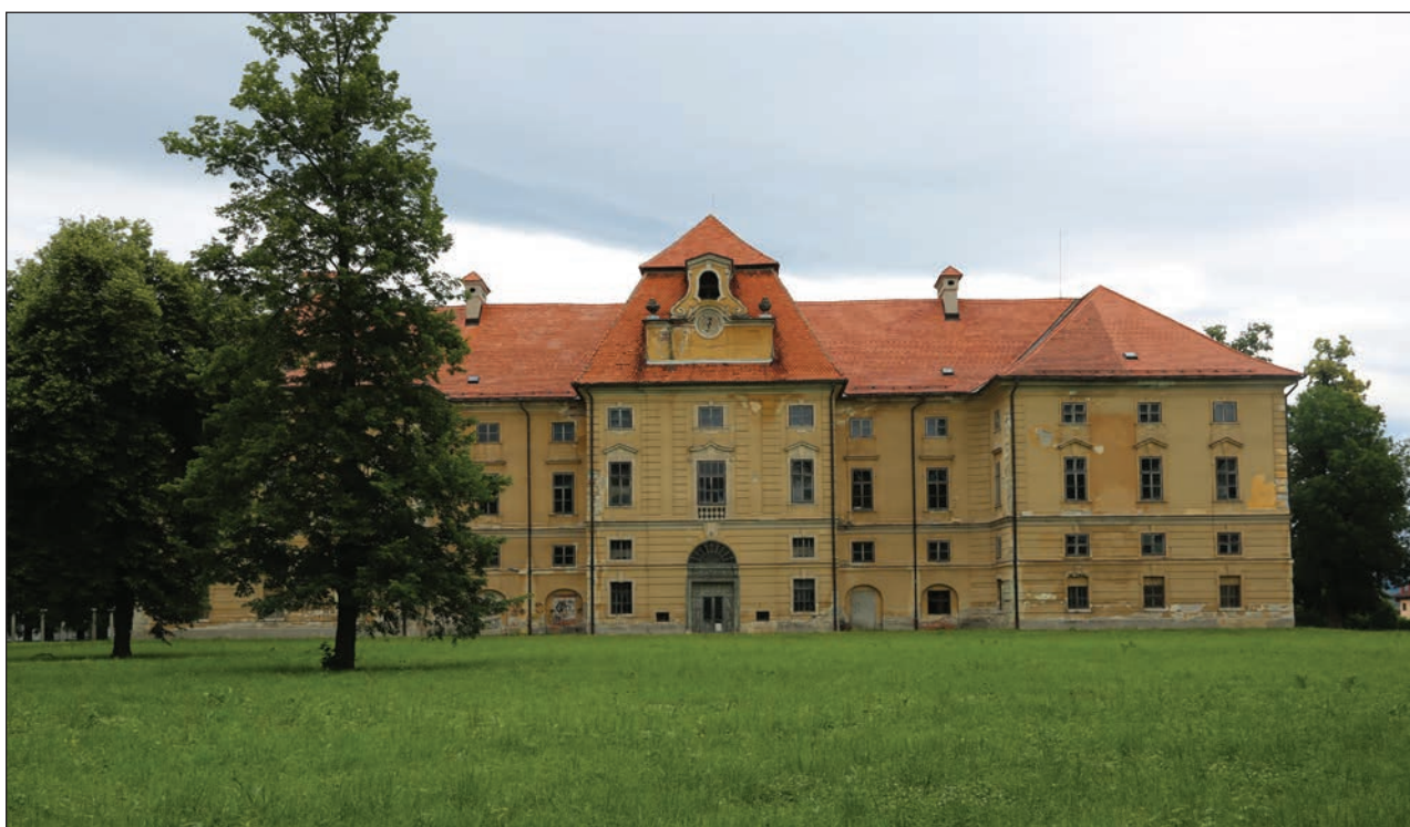
Figure 22: A view of the rear facade of the Novo Celje manor, 2020 (Photo: I. Sapač).
