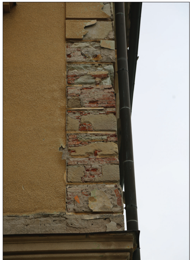
Figure 11: On one of the corners of the manor, older building elements processed by stonemasonry are used as a spoliation, 2022 (Photo: I. Sapač).
