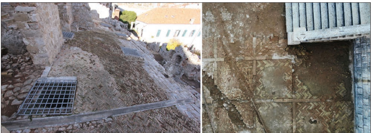
Figure 14: Brick pavements in the heringbone style (opus spicatum): area of the communal granary (Na Andriji); in front of the church St Blaise (Photo: ARHEO PLAN d.o.o).
