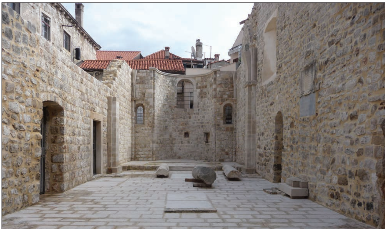
Figure 3: Remains of the church of St Stephen on Pustijerna, A.6 (Photo: Antun Baće).
