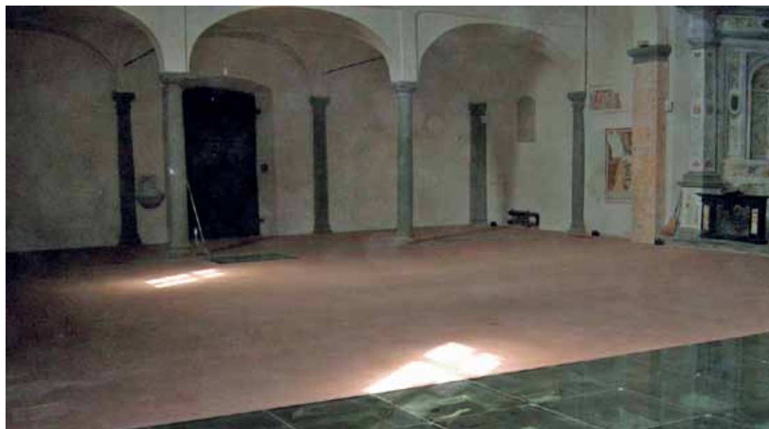
Fig. 19: Santa Maria del Lavello, the new pavement, partially opaque and partially realized with supporting glass tiles (Courtesy of G. Cruciani Fabozzi).
